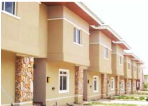
Electrical and Mechanical Services, Plumbing, A/C Installation Services Dove Court Phase 2, Utako District Abuja.
